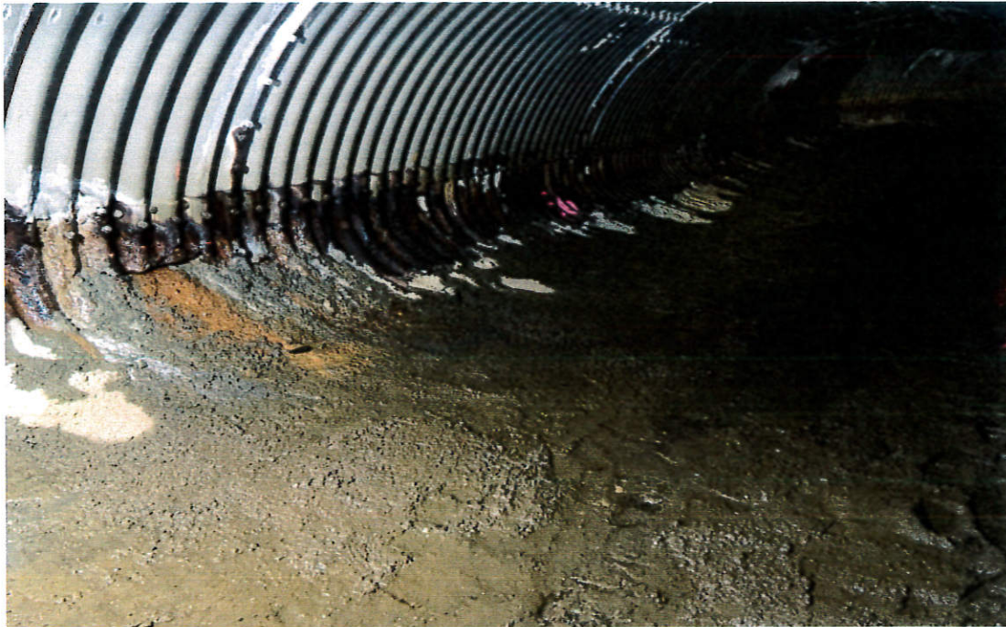
Schoenbar Culvert after Temporary Concrete Placement
